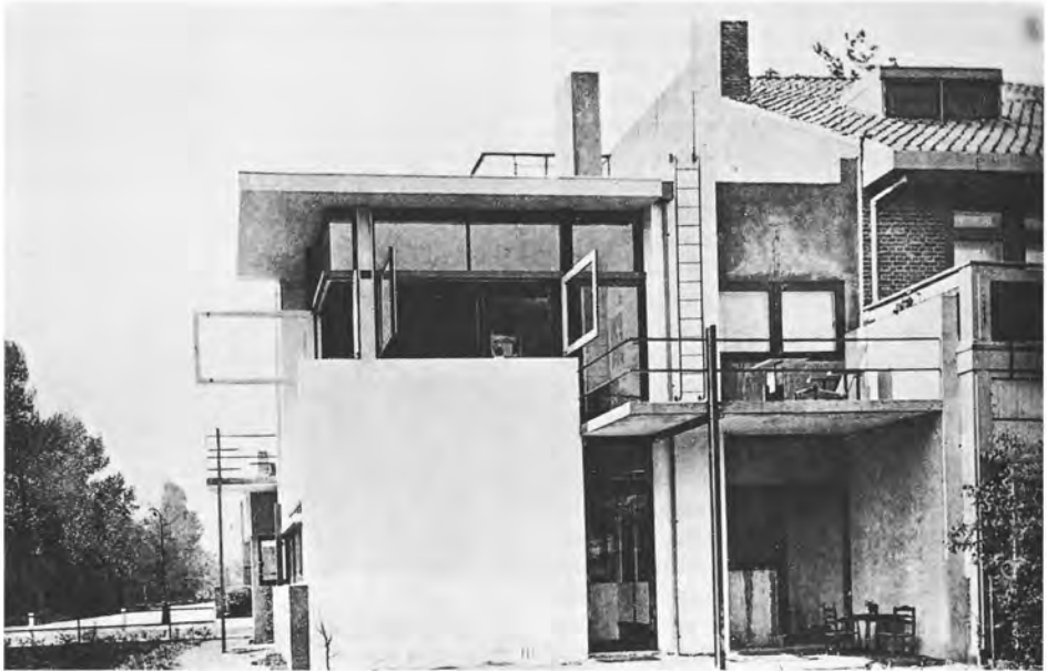
129, 130 Rietveld, Schröder-Schröder House, Utrecht, 1924. Right , plans of the upper floor, 'closed' (above) and 'open'.
