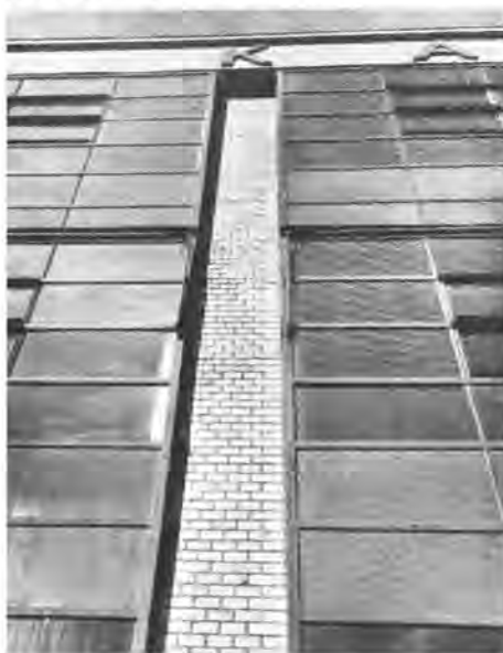
92 Gropius and A. Meyer, detail of the Fagus Factory, Alfeld-an-der-Leine, 1911.
