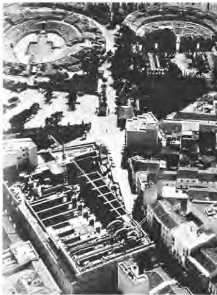
356 Moneo, National Museum of Roman Art, Mérida, 1980–85. Air view of the museum under construction showing its relation to the town centre and Roman amphitheatre and theatre.
