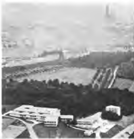
287 Bill, Hochschule für Gestaltung, Ulm, 1953–55, showing (left to right) workshop block, library, administration building and student housing. In the distance is Ulm Cathedral.
