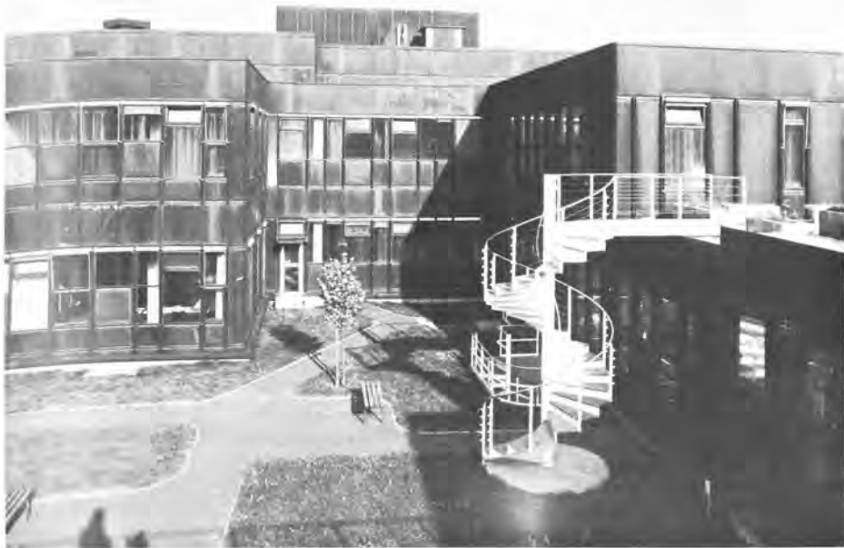
277 Woods and Schiedhelm, Free University, Berlin-Dahlem, 1963–73. Corten steel cladding system, detailed by Prouvé.
