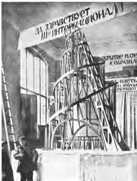
153 Tatlin, model of monument to the Third International, 1919–20. Tatlin stands in the foreground, pipe in hand.
