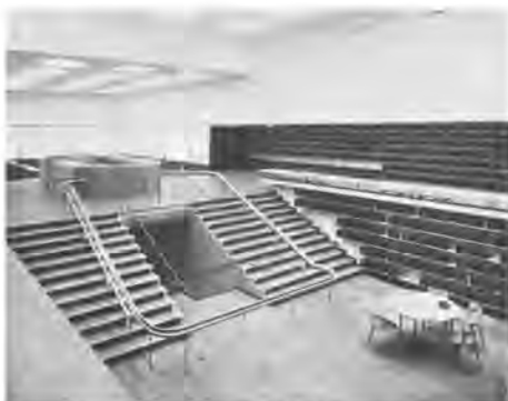
186 Aalto, Viipuri Library, 1927–35. Lending department, and reading room at higher level.
